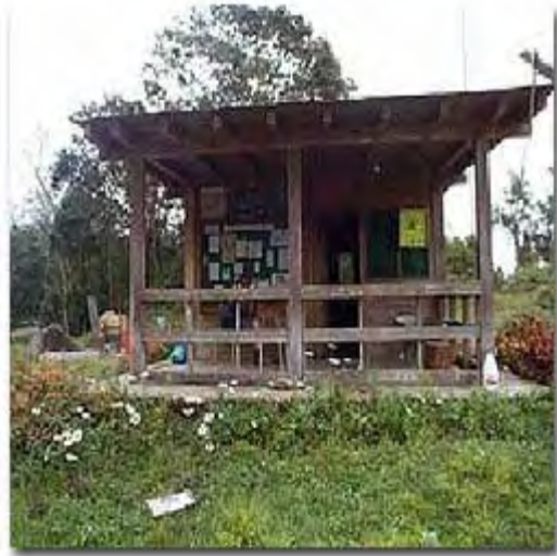
The old ranger station located at El Blanquito remains in shambles (Photo: César Aponte during the first park visit in 2001)
