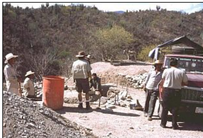
Construction of guard stations
