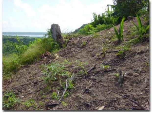
Steep slopes: erosion
