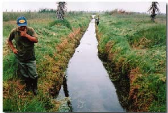
Maintenance of drainage canals
