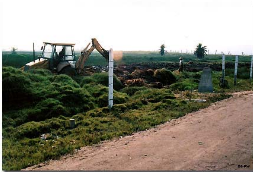
Digging a ditch around the protected area
