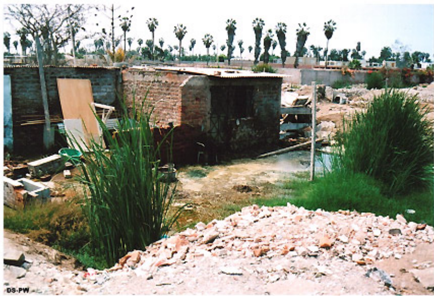
Flooding of houses in low plots
