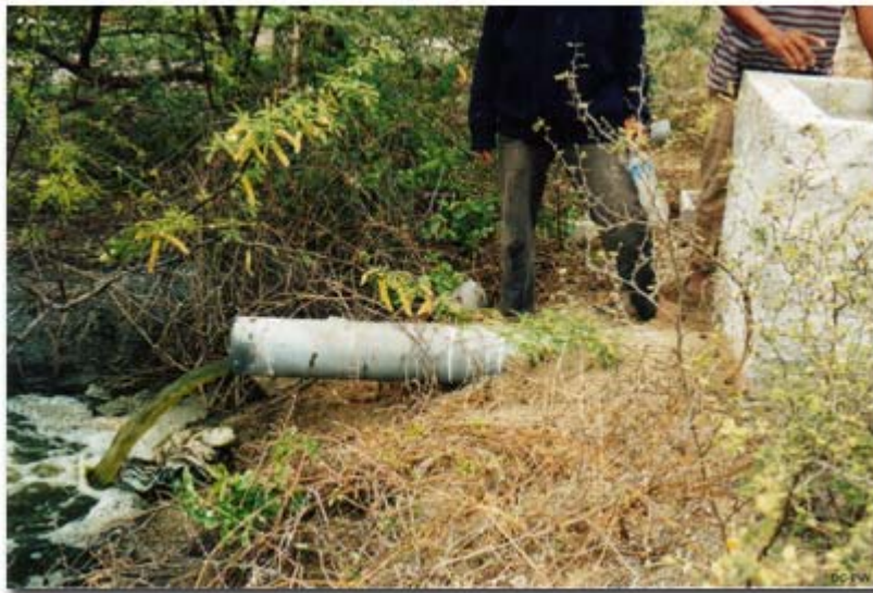
Effluents discharging directly into the environment. Photo: DS.
