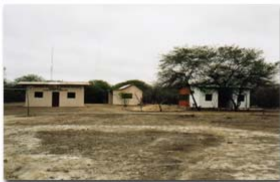
Control Station in El Algarrobo. Photo: DS.
