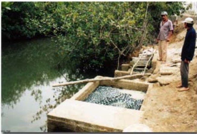
Effluent collection – these discharge straight into the water
