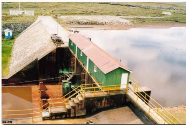
Upamayo Dam in the northern section of the lake
